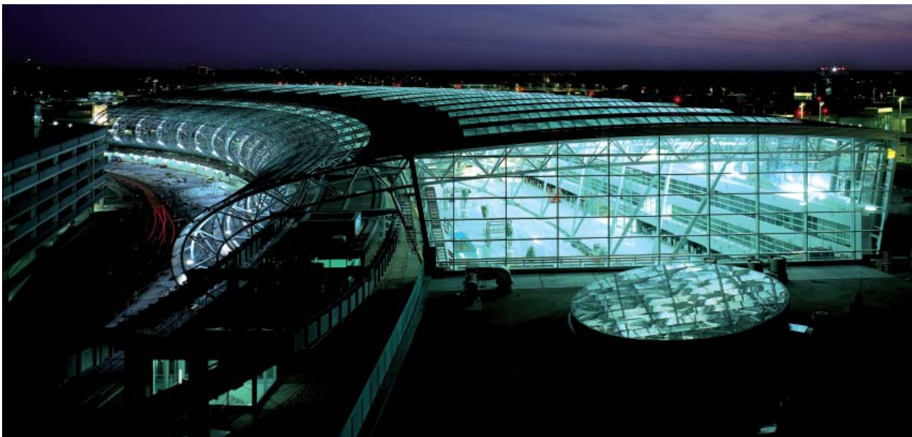
Fig. 3. The round-the-clock operation of airports imposes tough requirements on the control gear used – QTP8 units are ideally suited to such demanding applications
